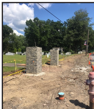
Sidewalks removed and new stone pillars
